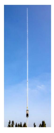
Install vertical antenna to the existing isopole antenna mast on elevator machinery room atop Edgewood building
